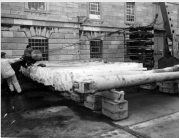
Gun barrels being stacked with pulleys in Melville Courtyard
