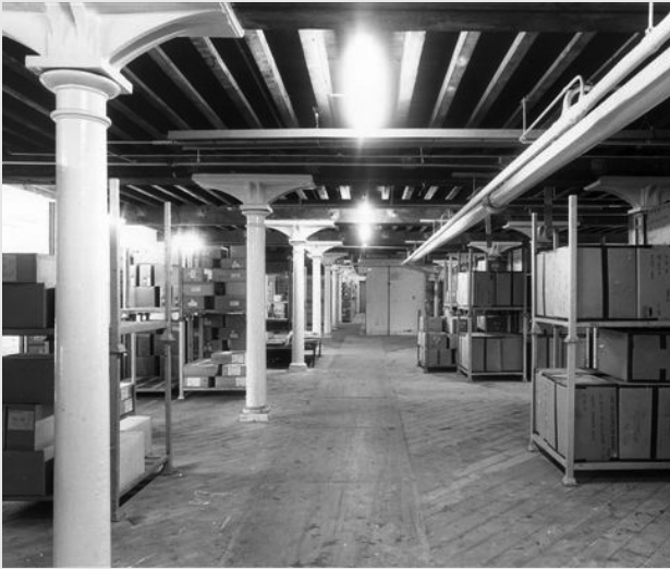
Storage in the ground floor of Melville
