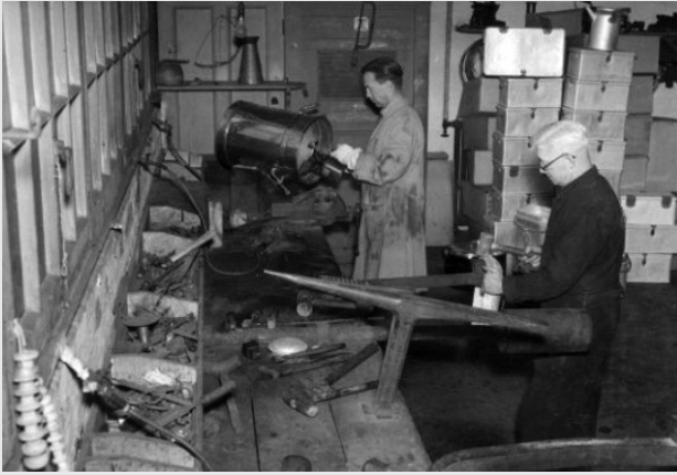
Repairing Tea Urns
